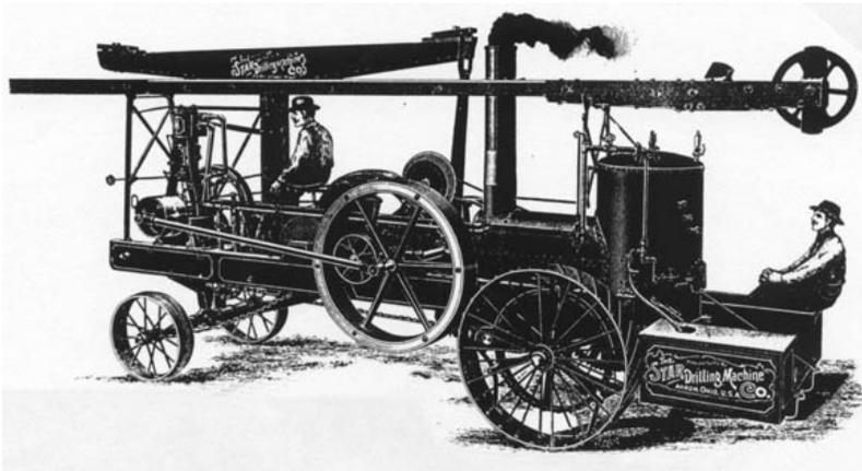
Star No. 2 or 800 foot drilling machine with traction attachment. It has a T shaped boiler. The vertical steam engine is at the front. The machine has a mast and a walking beam. Circa 1910
