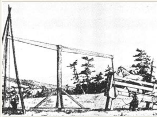
*This horsepowered treadle is rigged to a wooden walking beam rather than a spring pole. This arrangement was in use in the early salt days and also served for drilling shallow water wells. This cable tool rig is considered portable. Ca. 1810.*
